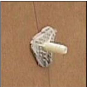
The epoxy capping material is applied over the crack to retain the injected resin. At the same time, additional resin is applied over the base of the pedestal. The epoxy resin is the same for both applications (setting the pedestals and capping or sealing the crack).
